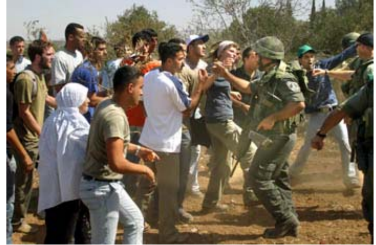
September 27, 04- Israeli border policemen scuffle with Palestinian and International demonstrators at the construction site of Israel's controversial separation barrier in the West Bank village of Beit Aawa near al-Khalil (Hebron)-
